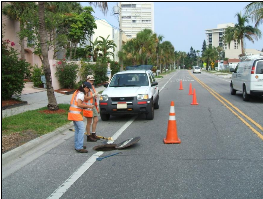
SKD-L Manhole at 312 Beach Road
