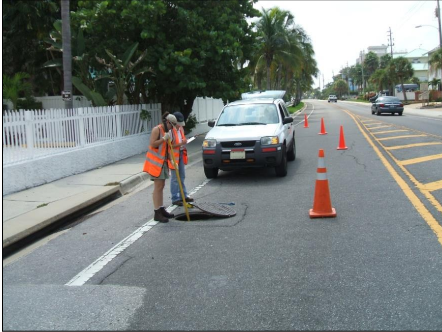
SKD-K Manhole at Beach Road and Calle del Invierno
