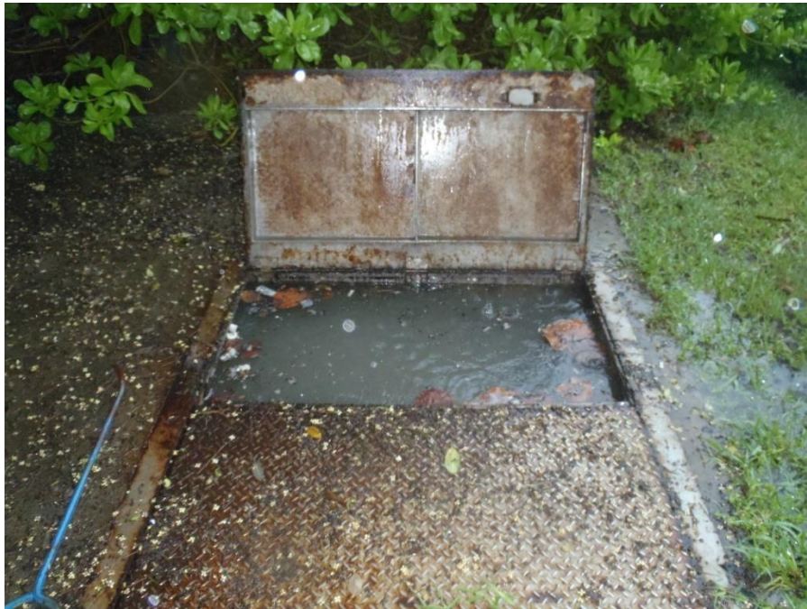
SKD-V Stormwater Vault during Tropical Storm Andrea 6-6-2013
