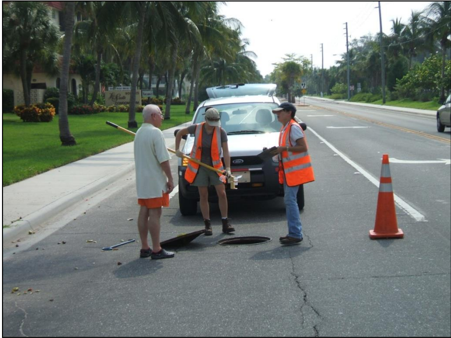
SKD-O Manhole at Beach Road and Beach Way
