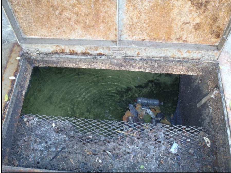
SKD-V Stormwater Vault - Normal Condition
