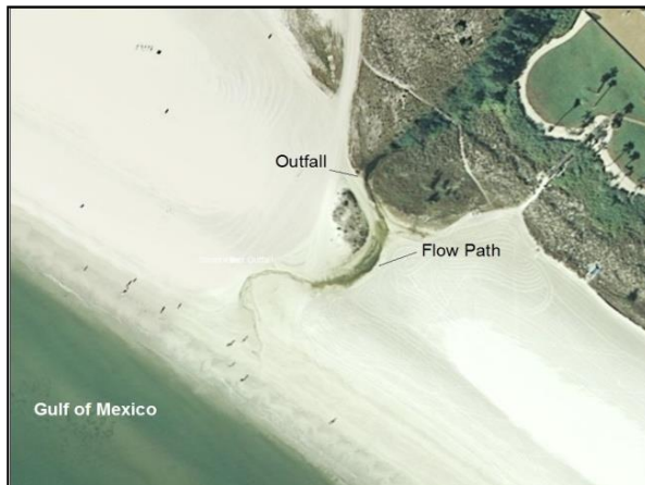
5-Outfall and Flow Path to Gulf Aerial
