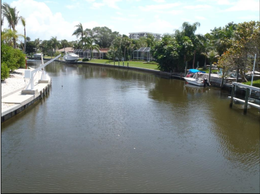
SKD-Q Grand Canal at Azure Road Bridge
