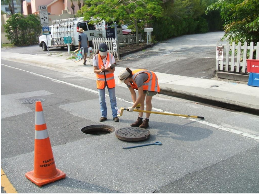
SKD-M Manhole at 460 Beach Road
