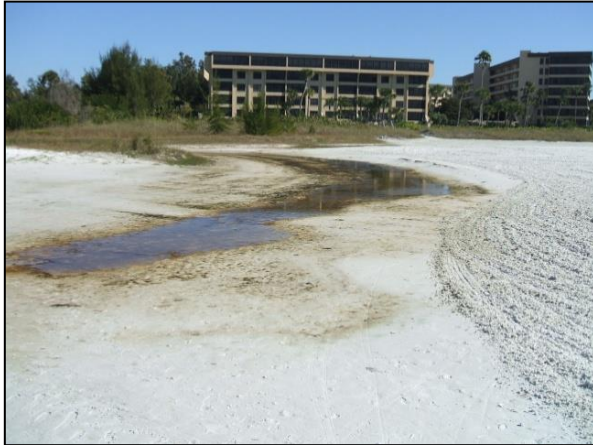
3-Flow from Outfall to Beach 1-25-2008
